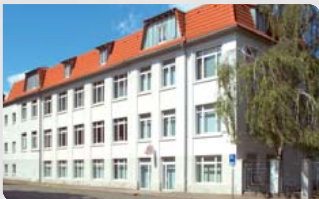
company building Schlegel Elektrokontakt GmbH, Leipzig
